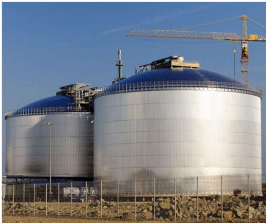
Fig. 1. Vertical storage oil tank [11].
