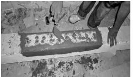
(c) Finishing Surface of beam soffit after fastening Ferrocement Laminates with the connectors
